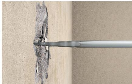
Chiseling in concrete wall
