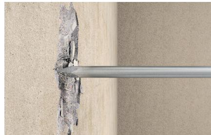
Chiseling in concrete wall
