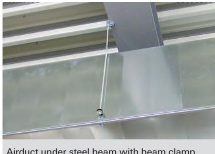
Airduct under steel beam with beam clamp
