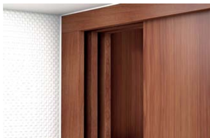
Wall connection joints
