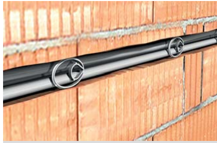
Cable fixing in wall slots > 30 mm
