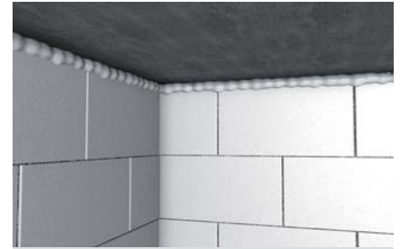
Closing joints in structural work
