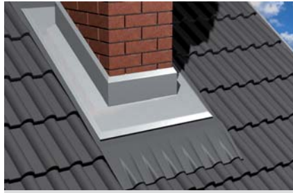
Sheet metal coverings
