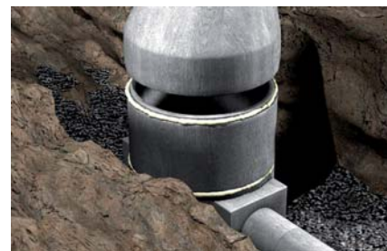
Sealing concrete manhole rings
