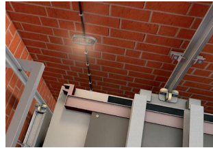
Elevator guide rails
